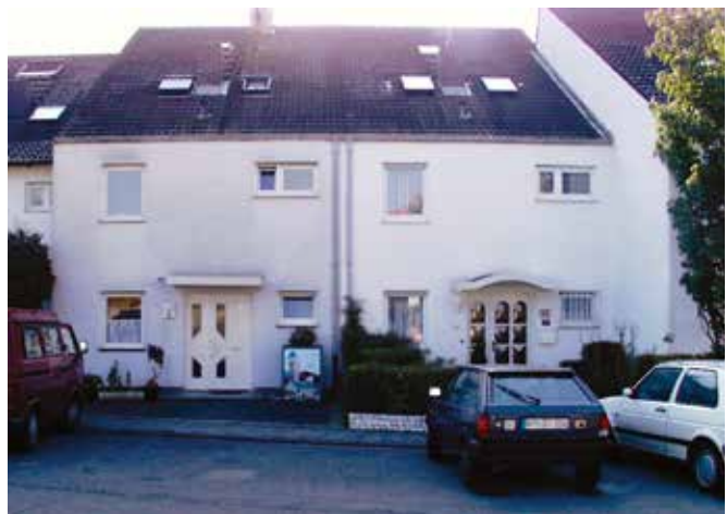
Figure 3 Facade of a duplex house after a period of eight years Duplex house left: Paint without SIPERNAT® 820 A Duplex house right: Paint with 5 % SIPERNAT® 820 A
